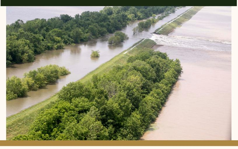
The U.S. Federal Emergency Management Agency (FEMA) defines a levee as a "man-made structure, usually an earthen embankment, designed and constructed in accordance with sound engineering practices to contain, control, or divert the flow of water so as to provide protection from temporary flooding." Levees are sometimes referred to as dikes.
